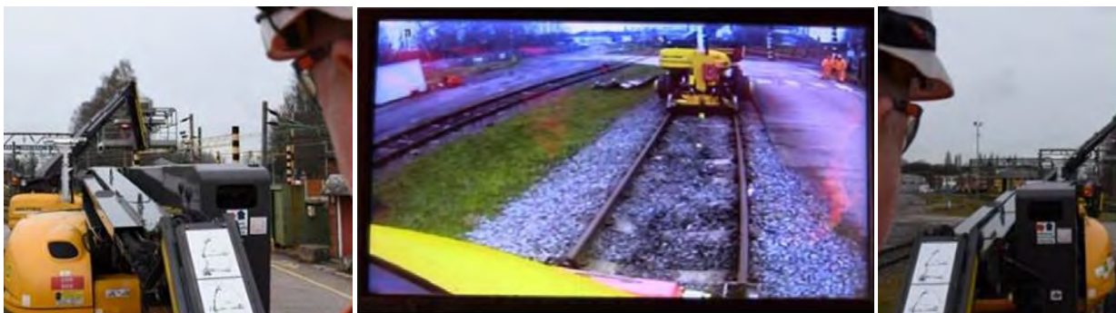
Figure 11: Images taken from MEWP 10, 15 metres from stationary MEWP 3, showing the view from the machine operator's eye level (left), CCTV monitor view (middle) and machine operator eye level view (right) from MEWP 10
