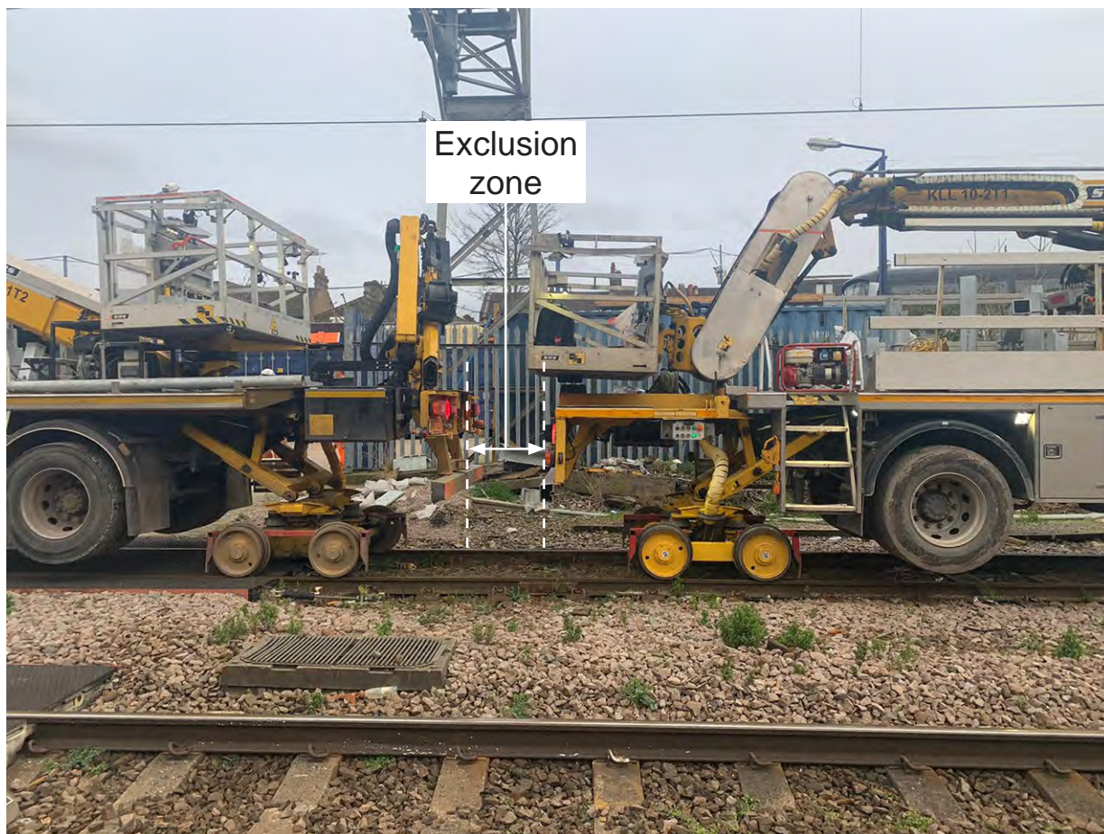
Figure 14: Image showing where the COSS was injured at Manor Park
