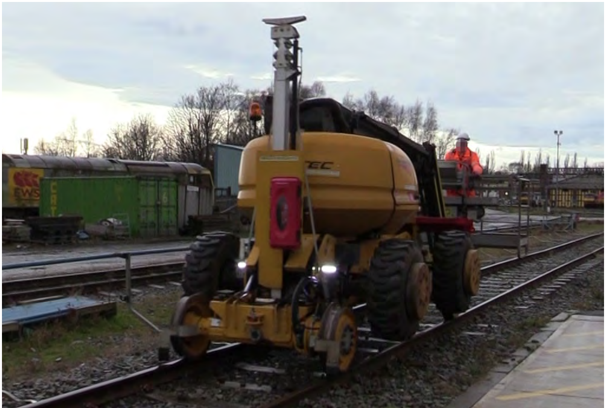
Figure 5: Skyrailer MEWP 10 involved in the accident
