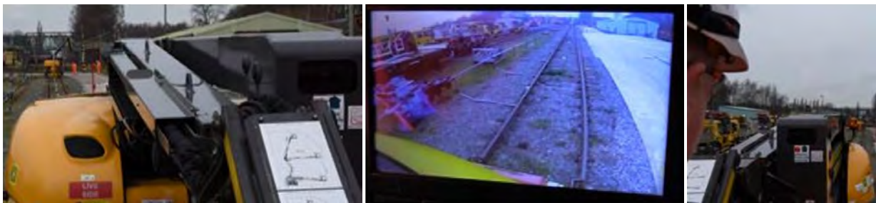
Figure 10: Images taken from MEWP 10, 107 metres from stationary MEWP 3, showing the view from the basket (left), CCTV monitor view (middle) and eye level view (right) from the machine operator's perspective on MEWP 10
