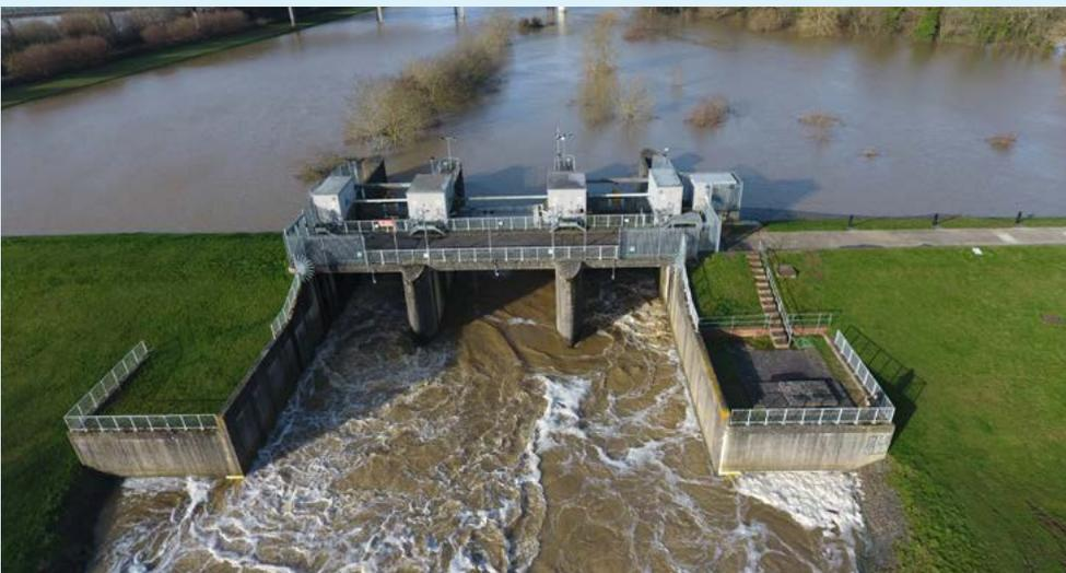
Figure 21: Leigh Flood Storage Area in operation, Kent.
