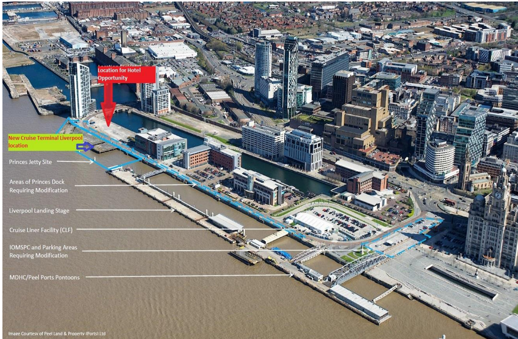
Figure 1: Development area (image courtesy of Peel Land and Property (Ports) Ltd – provided by Liverpool City Council)
