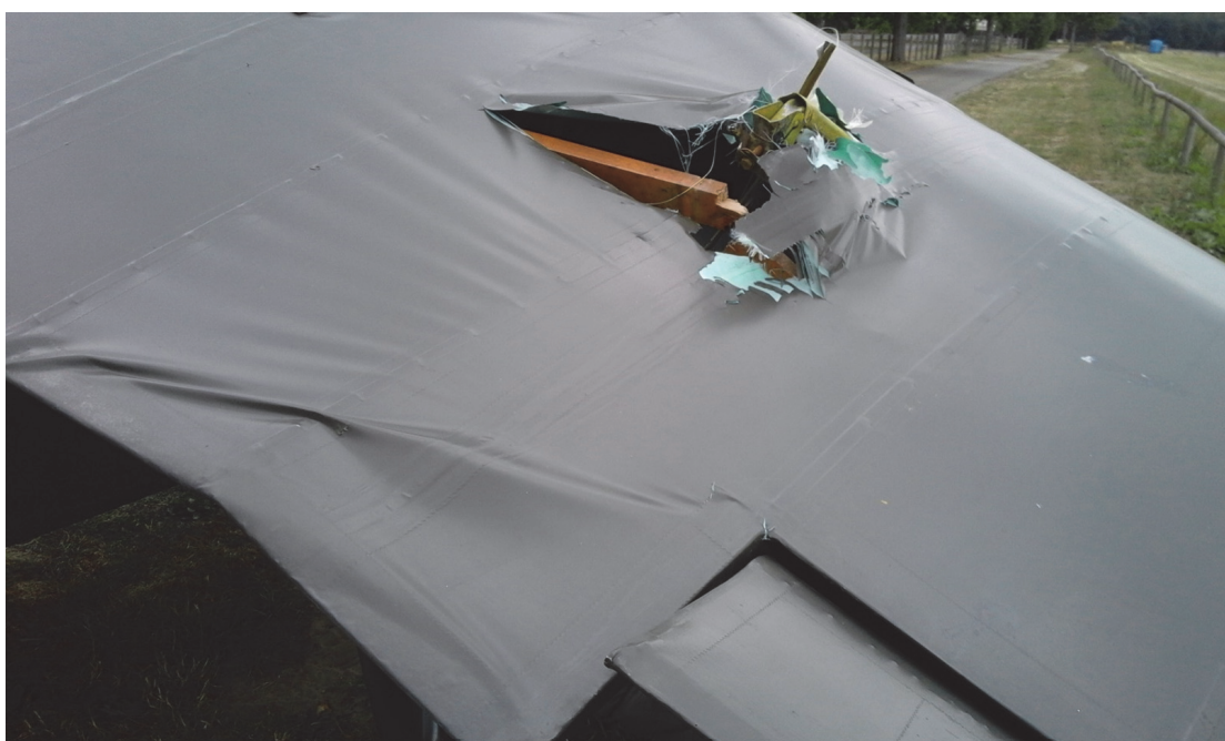
Figure 2 Damage to the right wing
