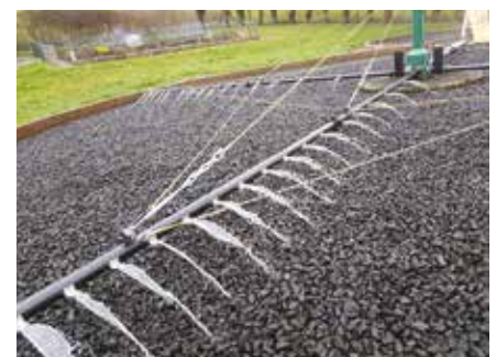
The new filter arms on the sewage treatment works © Ancala Water Services
