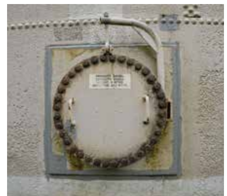
Typical 24" access hatch at base of tank © Crown
