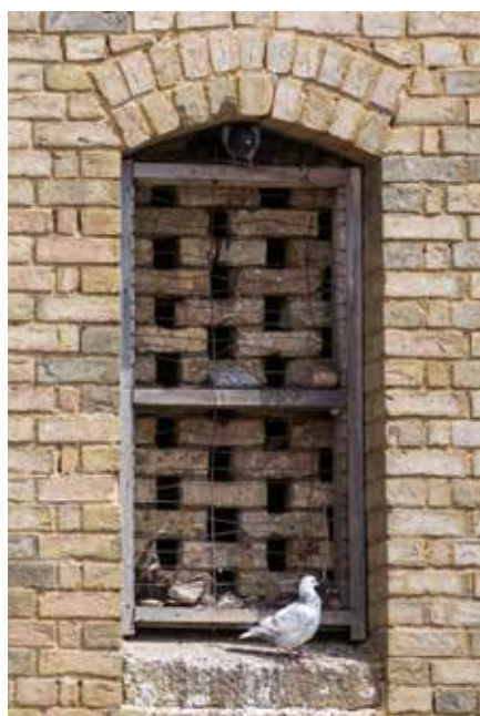
The re-pointing works completed at Martello 14 © Landmarc Support Services
