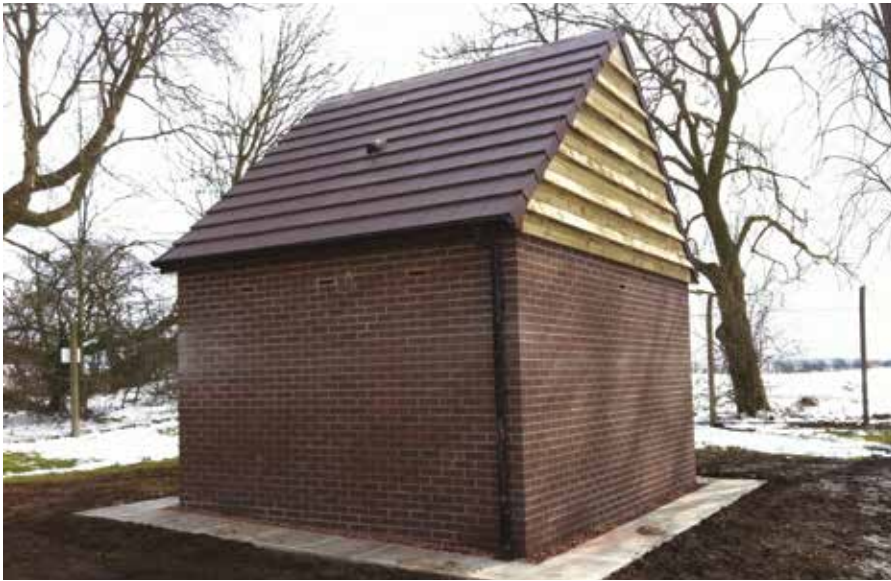
Bat house – built with cavity wall and loft space to mitigate the demolished building © Crown
