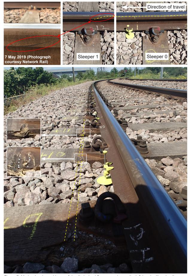
Figure 7: Marks showing evidence of derailed wheel flange running on the left-hand railhead, rail fasteners and sleeper ends (all photographs 23 May 2019, except as labelled)
