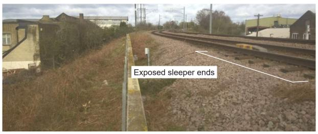
Figure 12: The condition of the up-side cess and ballast around 0 miles 27 chains on the up High Level lines as photographed during the specialists' site visit of 15 March 2019 (photograph courtesy SNC-Lavalin)
