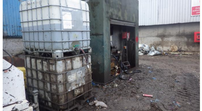
908 Liquid storage without secondary containment
