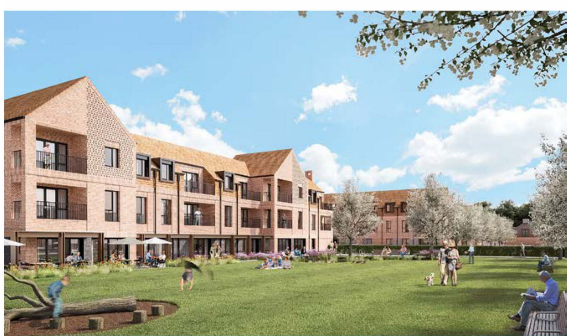
Mixed-use development at Burston Garden Centre St Albans, Hertfordshire
