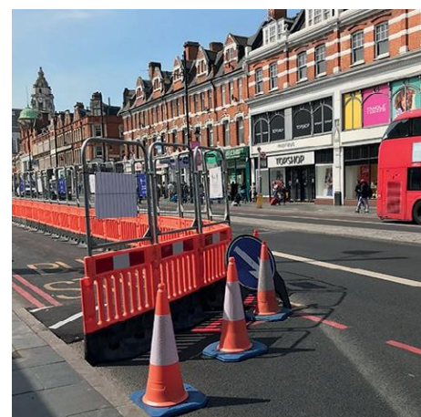
Figure 32: Footway widening outside station entrance – London
