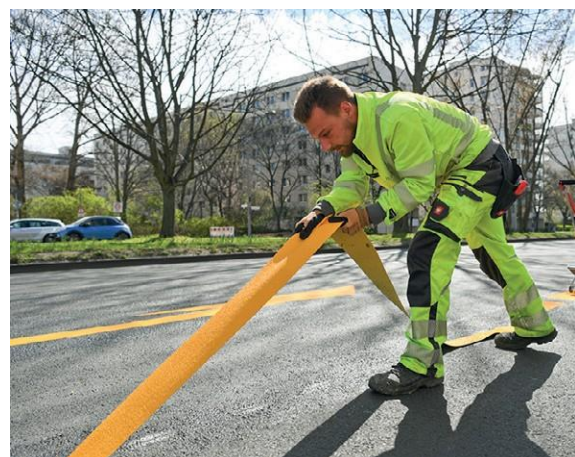
Figure 29: Pop up cycle lanes being installed. – Berlin (Copyright, Reuters images)
