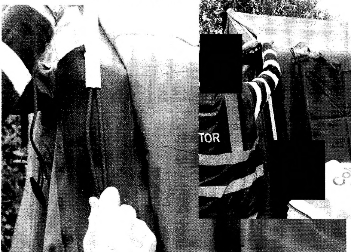
Figure 46: Installing wall keder using two (2) people
