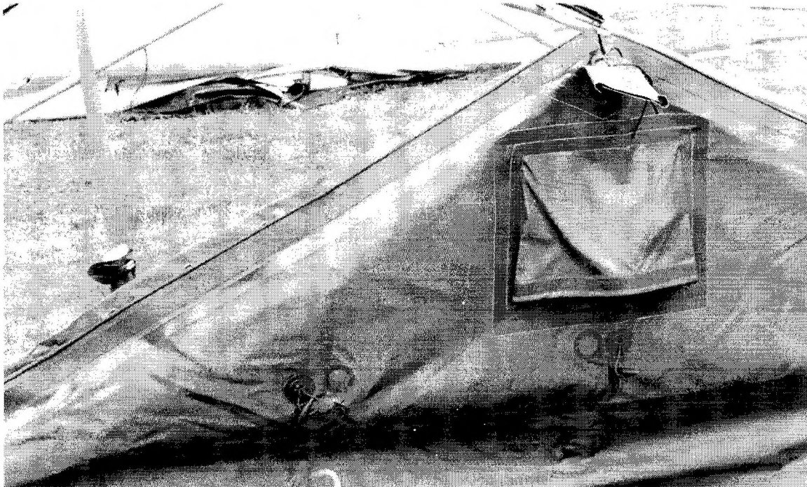
Figure 16: Installation of end gable strap with insets of hook connection
