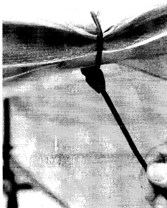
Figure 43: Tensioner Fitted
