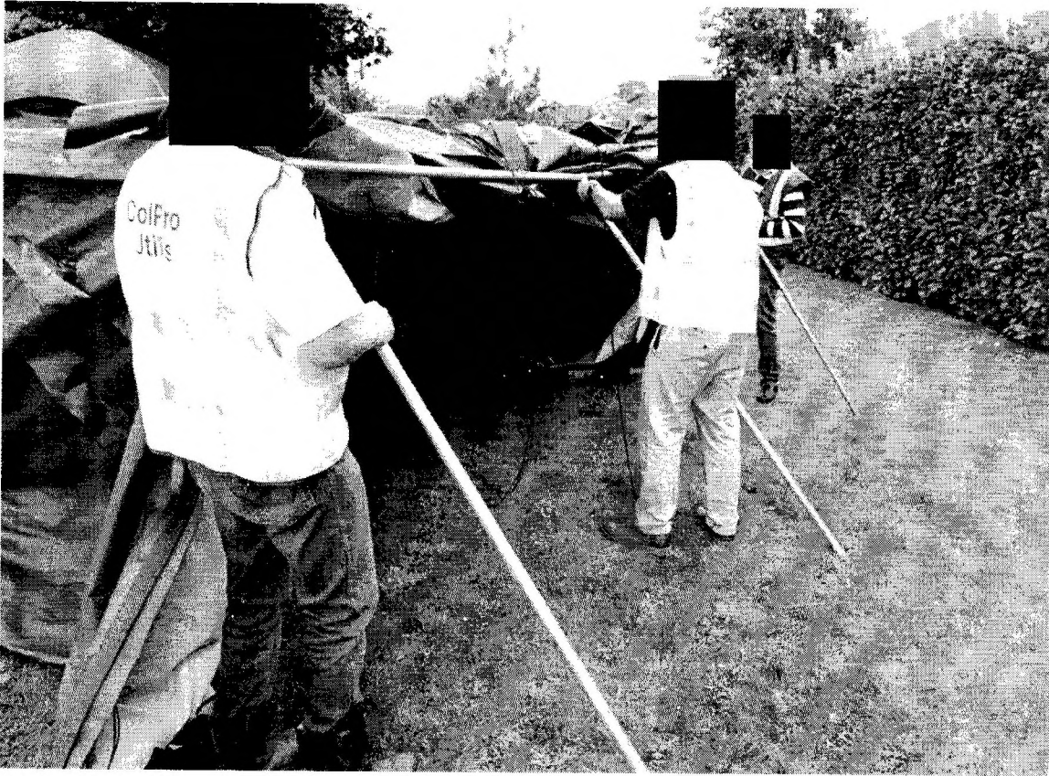
Figure 38: Shelter legs fitted on one side
