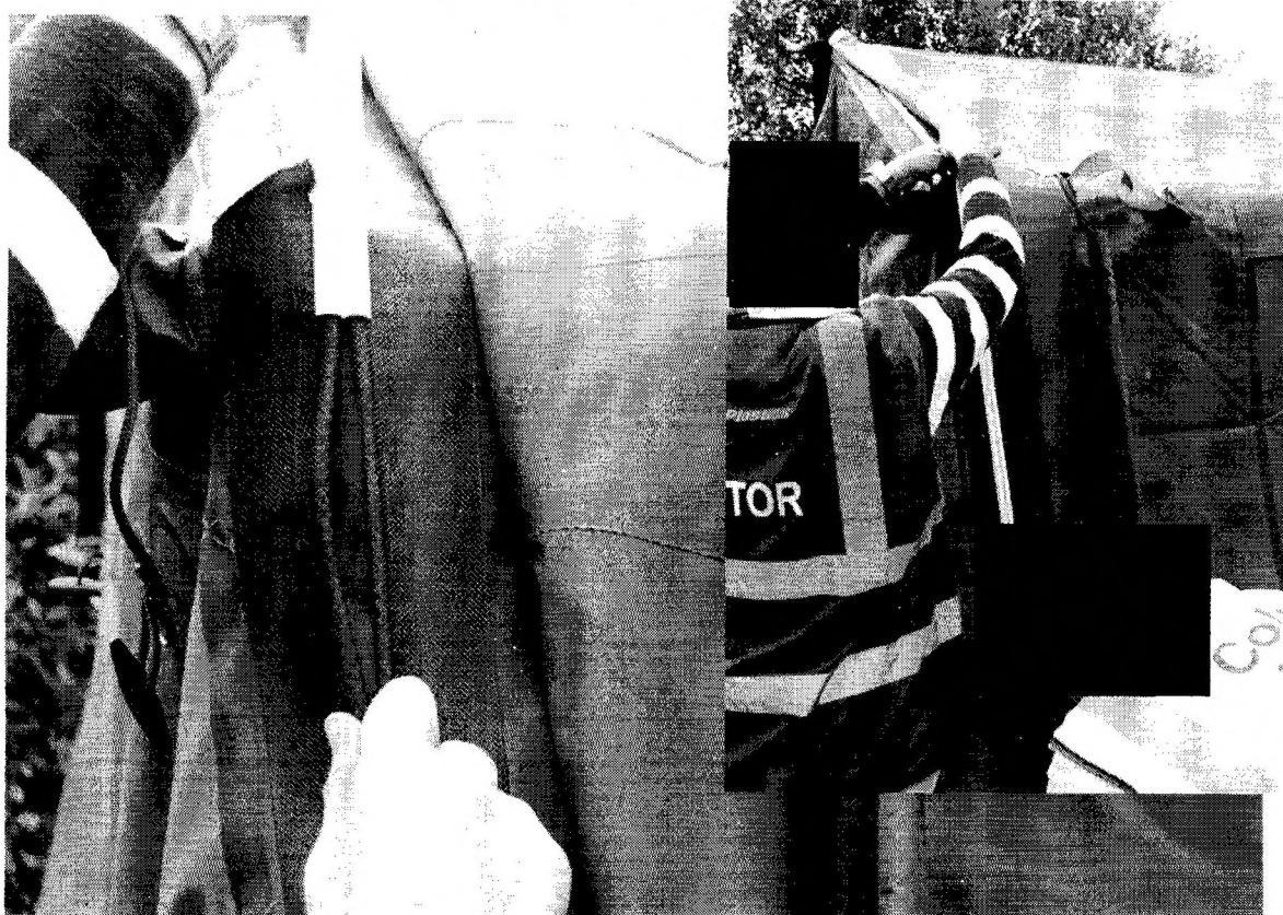
Figure 33: Installing wall keder using two (2) people (Passageway to tent or end wall)
