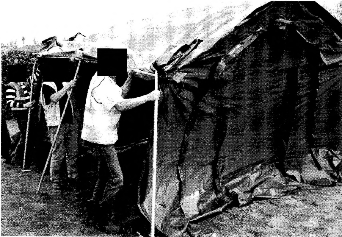
Figure 41: Install the legs on the other side of the tent
