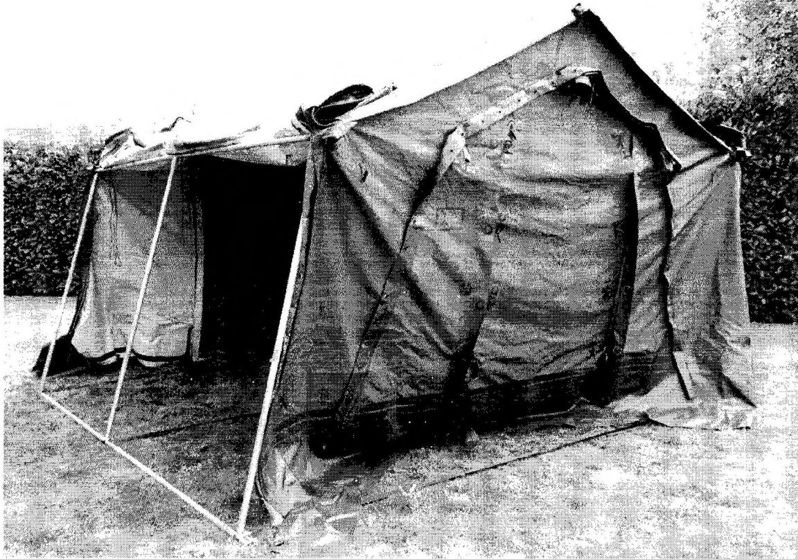
Figure 45: Tent ready for connecting side walls
