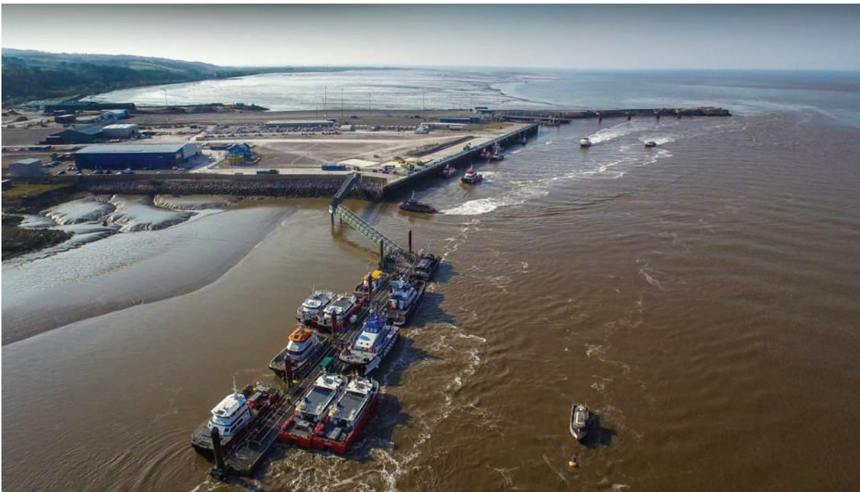
Figure 6: The Control Room is based at the O&M building, which is adjacent to the Port of Mostyn
