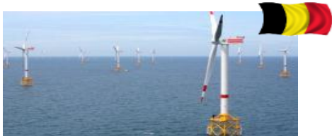
Thornton Bank I-III 2) , BE, 325 MW: Completely commissioned 2013
