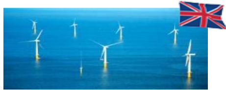
Rhyl Flats, UK, 90 MW: Completely commissioned 2009
