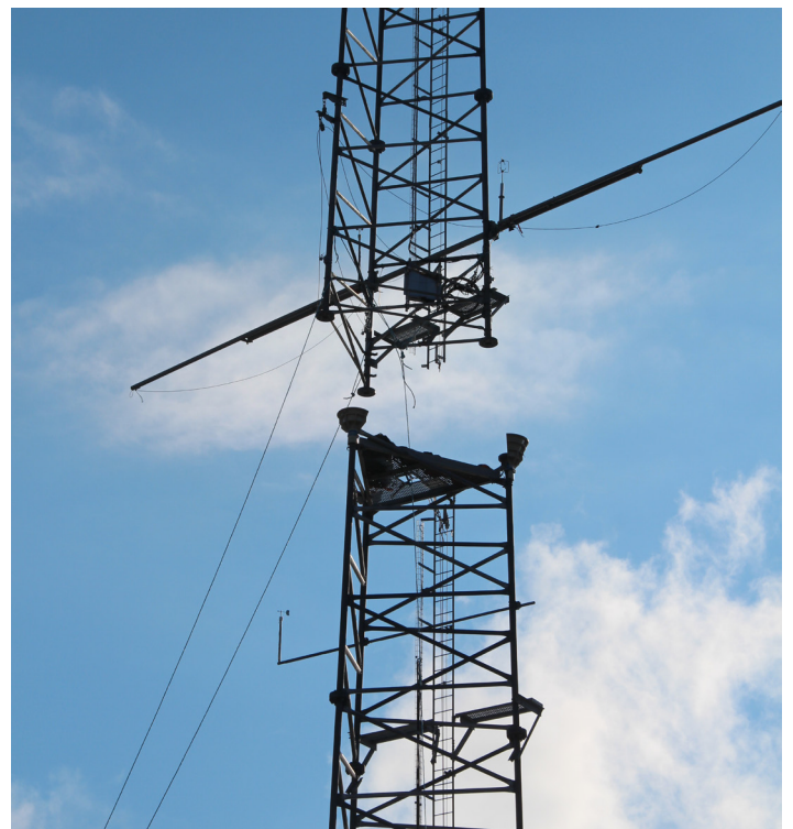
Landing the upper tower section with the use of guide cones and video cameras.
