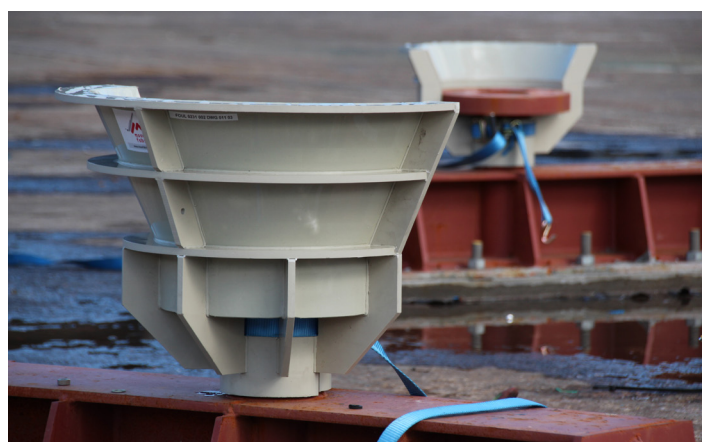
Plastic guide cones attached to the flanges.
