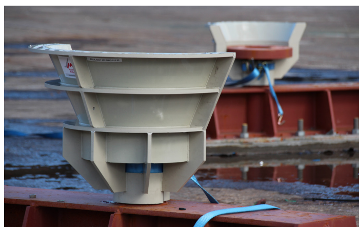
Plastic guide cones attached to the flanges.
