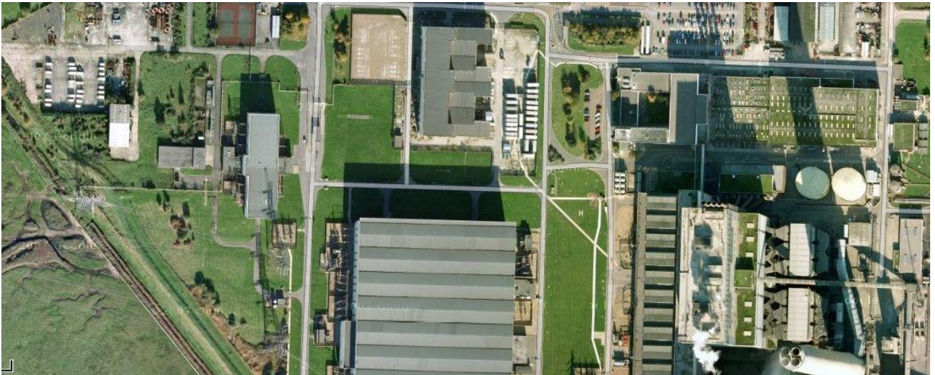
Figure 2: Aerial view of Kingsnorth 132kV Substation (top centre)
