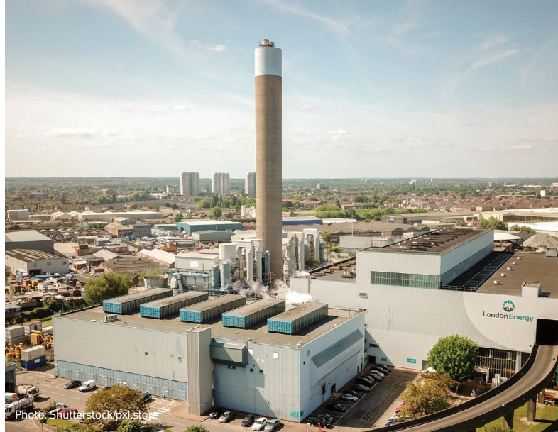
The North London Waste Authority is building a £500m replacement energy recovery facility at the Edmonton EcoPark in north London after winning Government backing. Construction work began in January 2019 and is expected to be completed by 2025. Our Plymouth Office registered the acquisition of an access road at the northern end of the site.
