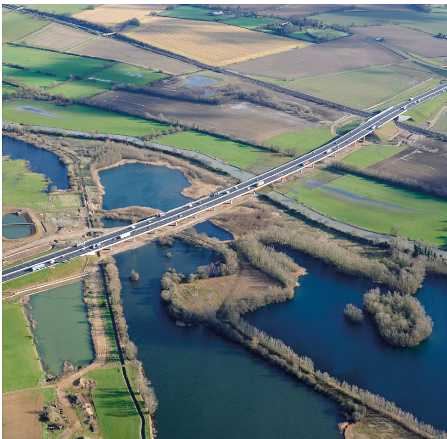
A14 Cambridge to Huntingdon improvement scheme, DfT
