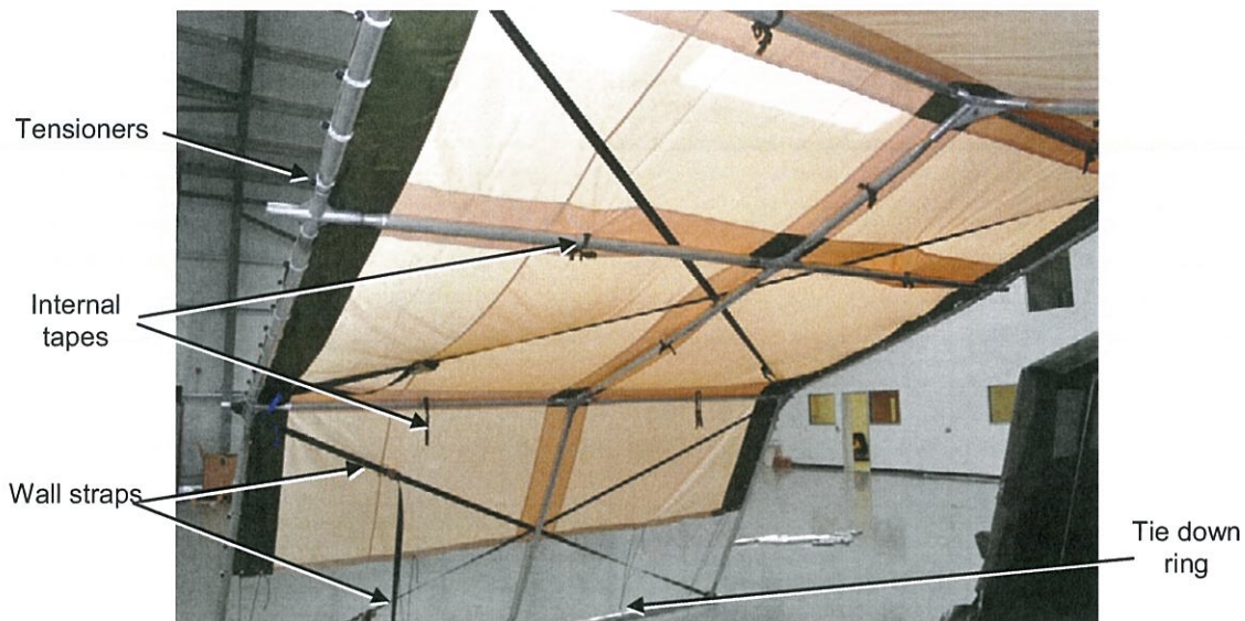
Fig 3 Attaching the cloth to the roof frame assembly
