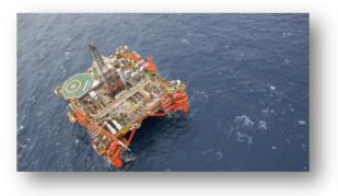
In the Don field, oil was discovered in the sandstone of the Middle Jurassic Brent Group in 1973. The discovery was subsequently appraised by Shell/ ESSO in 1976 and then developed by BP in the 1990s. EnQuest's redevelopment began production in 2009. The development consists of four sub-sea tie-backs: Don South West, West Don, Conrie and Ythan all tied back to the Northern Producer installation.
