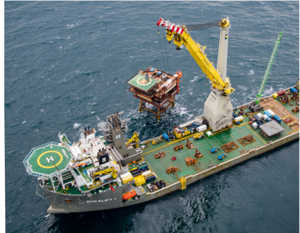
The Bokalift 1 working in the Southern North Sea
