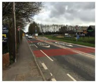
Figure 3-13: Faded advisory cycle lane, providing poor provision alongside 40mph traffic, Link 4
