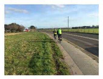
Figure 3-31: Narrow shared use path with poor surface quality, Link 9
