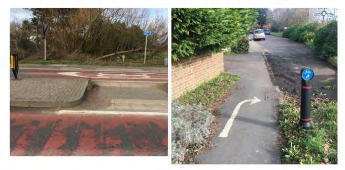
Figure 3-26: No cycle specific signage or provision across Station Road roundabout, Link 8
