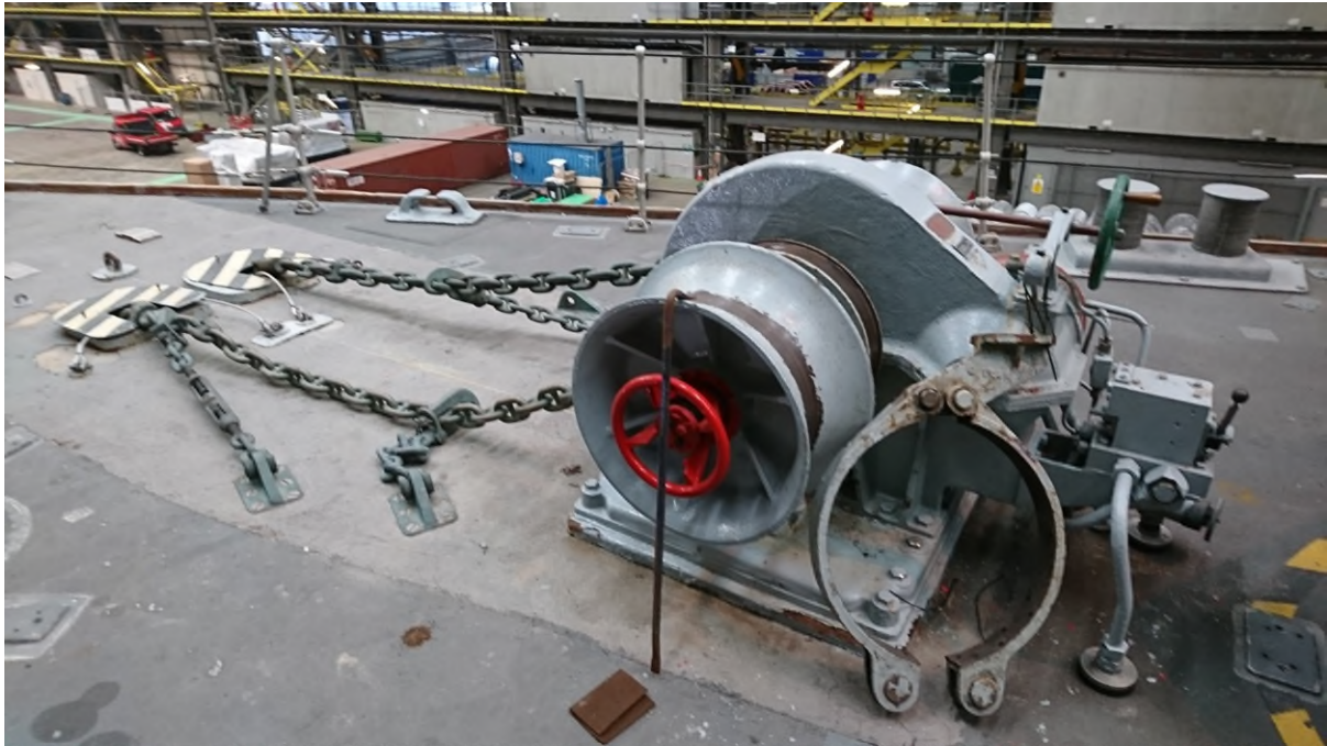
Focs'le anchor windlass and cable holder port. Note, only one set of cable and anchor will remain.
