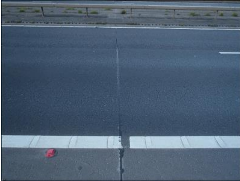
15 - North pier joint, Northbound
