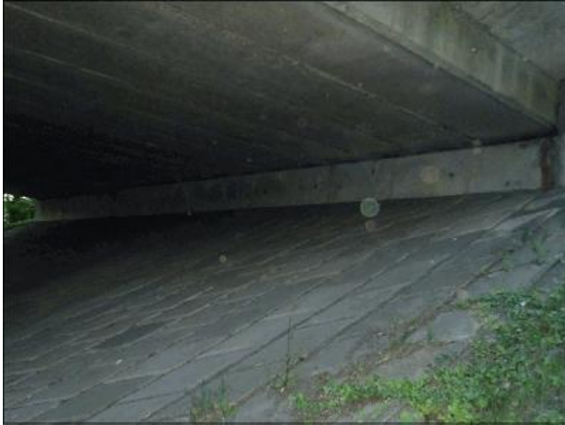
03 - North bankseat and revetment
