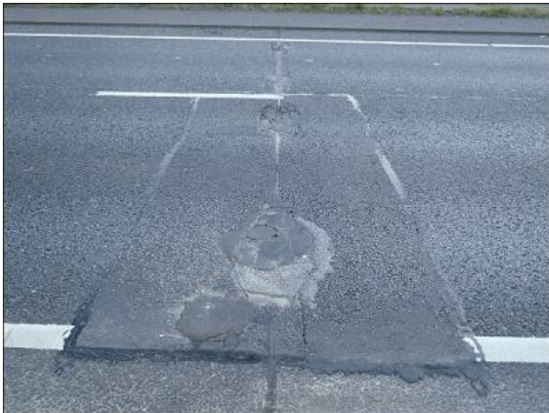
16 - North pier joint, Southbound
