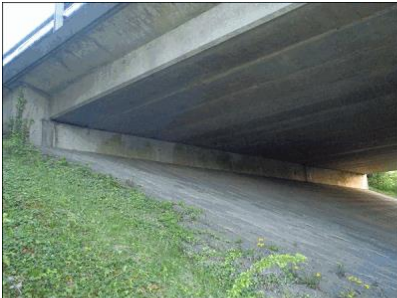
04 - South bankseat and revetment
