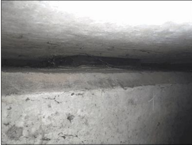
07 - Typical bankseat bearing, North
