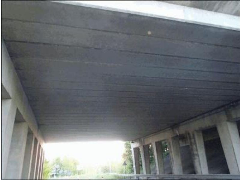
09 - Main span deck soffit
