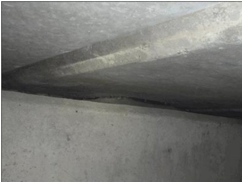
08 - Typical pier bearing, South
