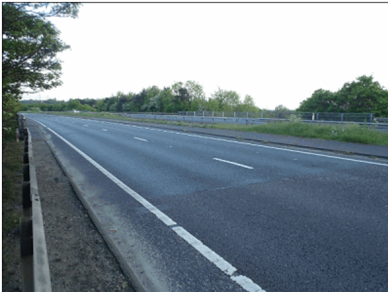
12 - View over Southbound carriageway
