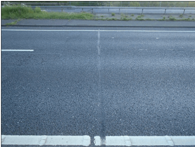
20 - South joint, Southbound
