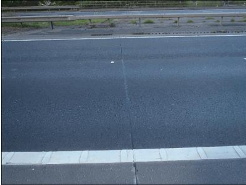
13 - North joint, Northbound
