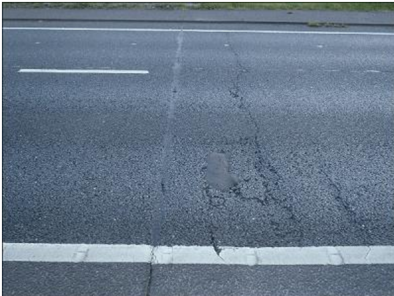
14 - North joint, Southbound
