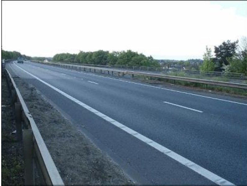
11 - View over Northbound carriageway
