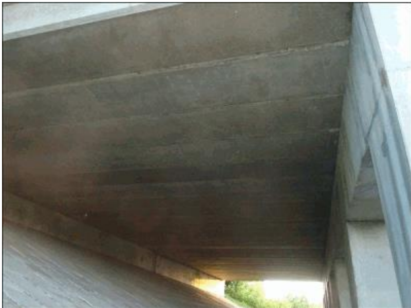
10 - South side span deck soffit
