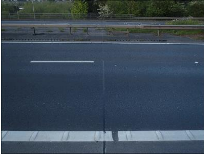
19 - South joint, Northbound
