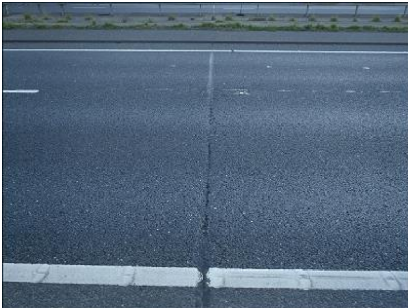
18 - South pier joint, Southbound
