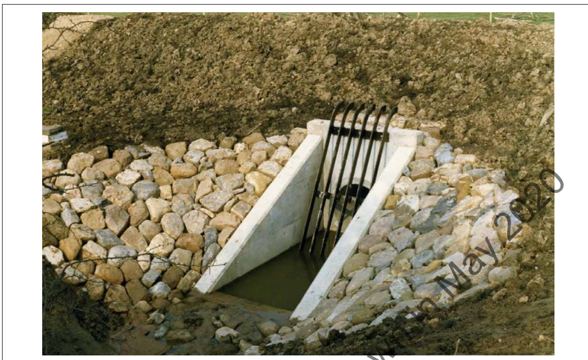
Figure 11.2 A debris screen on a small culvert.
