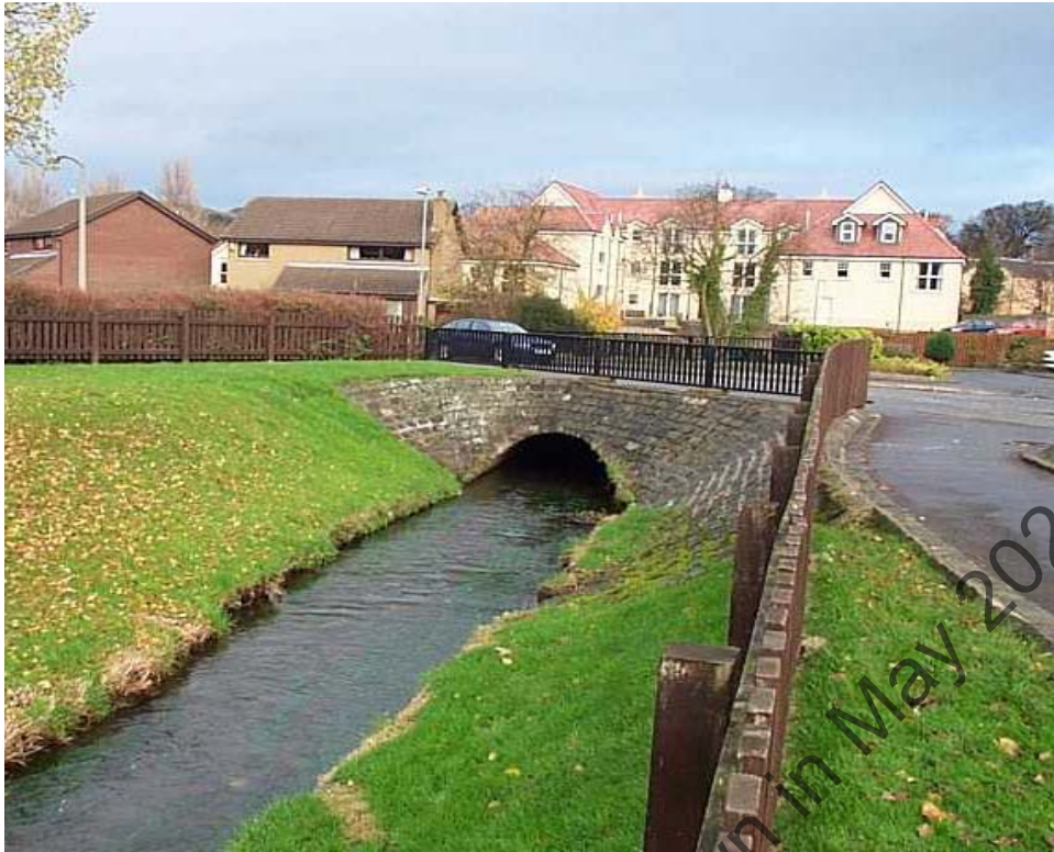
Figure 3.2 Culvert in a residential area with no requirements for a screen.
