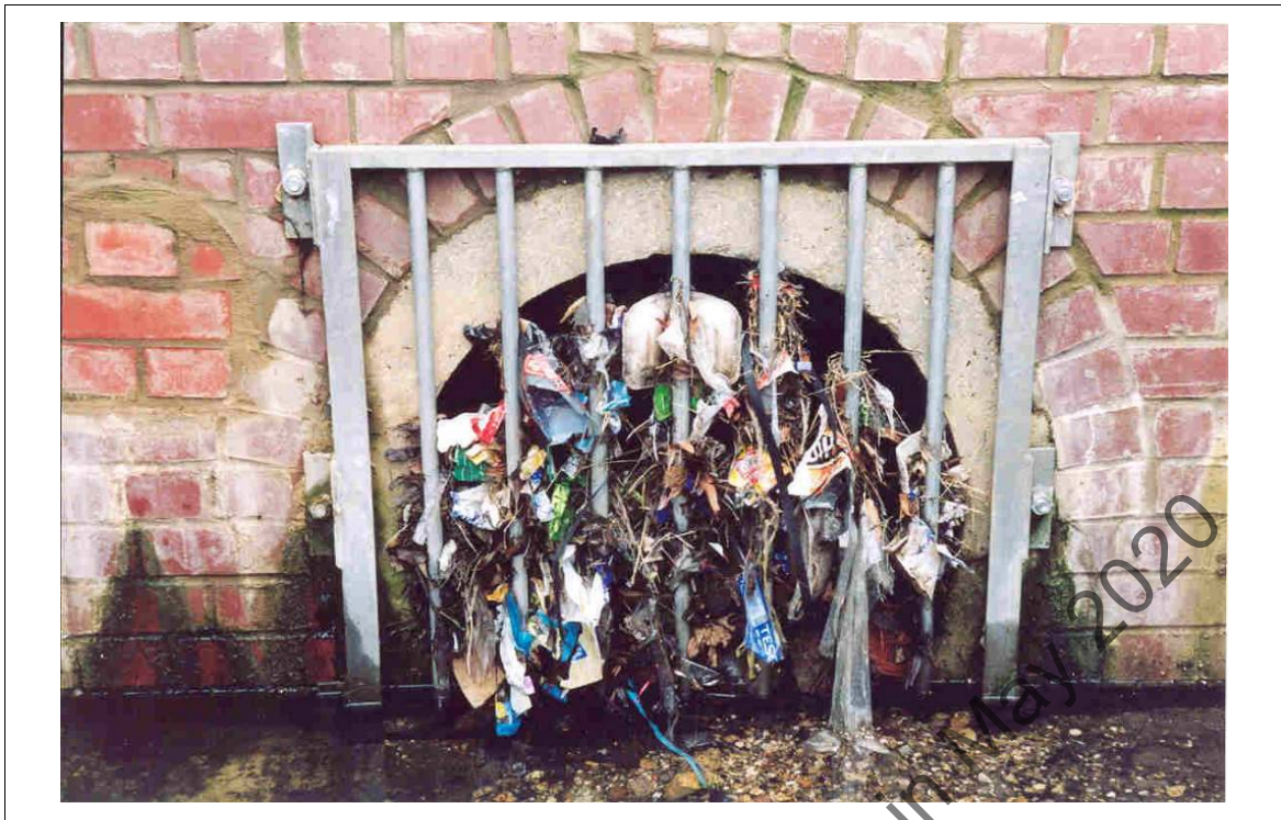
Figure 4.4 Crude security screen at the downstream end of a small culvert.
