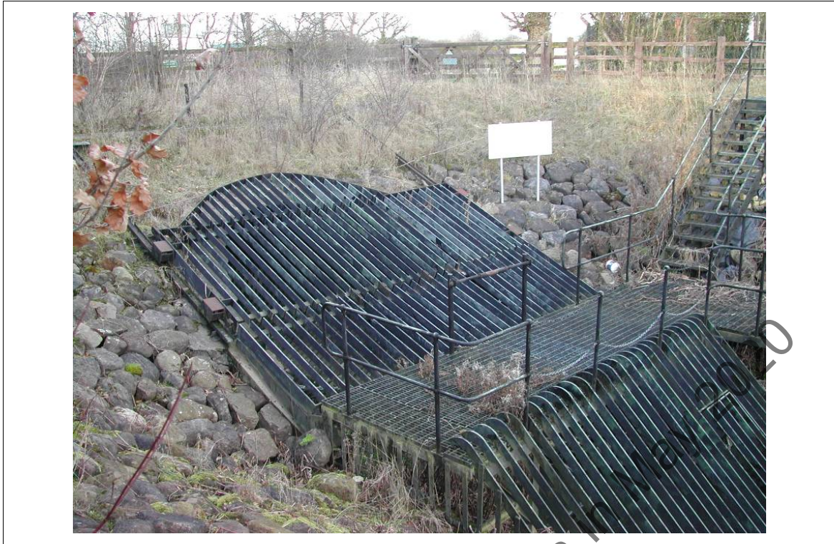
Figure 4.6 Security screen at the entrance to a large flood relief culvert.
