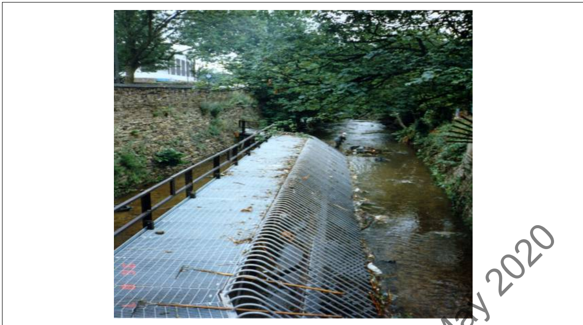
Figure 11.4 Screen on the River Sheaf with diagonal alignment to flow.
