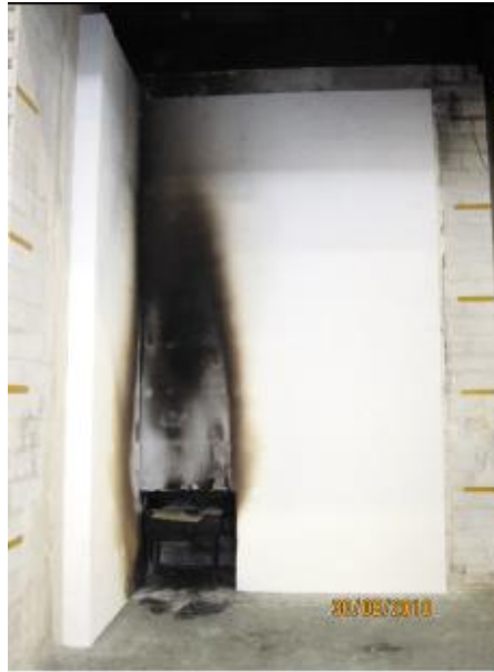
Figure A19 – External façade following test to DIN 4102-20 [52]
