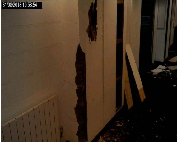
Intrusion 15 - Timber panel above link corridor doors
