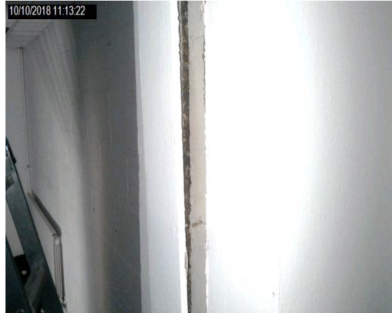
Intrusion 40 - Metal panels to foam to underside of external windows
