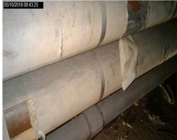
Intrusion 75 - Foil faced glass fibre insulation to metal pipework
