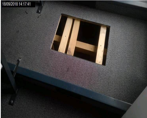
Intrusion 43 - Timber panel to block built riser
