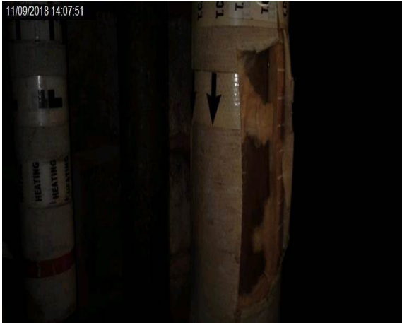
Intrusion 15 - Cloth wrap to glass fibre insulation to metal pipework
