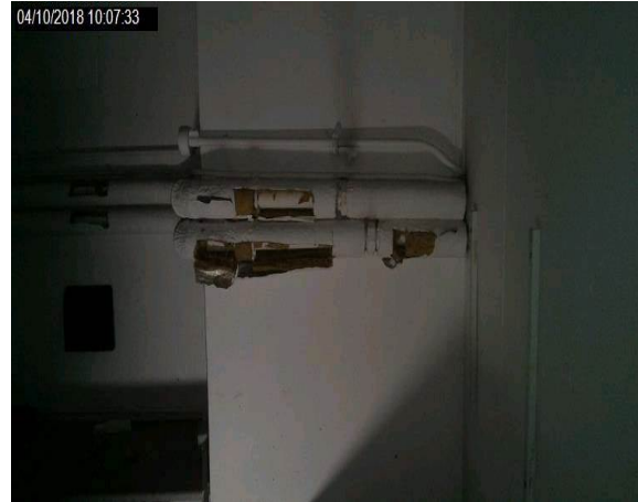
Intrusion 72 - Foil faced glass fibre insulation to metal pipework
