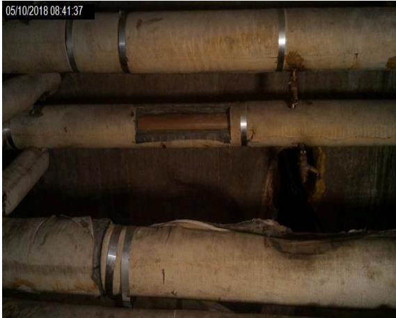
Intrusion 74 - Cloth wrap glass fibre insulation to metal pipework
