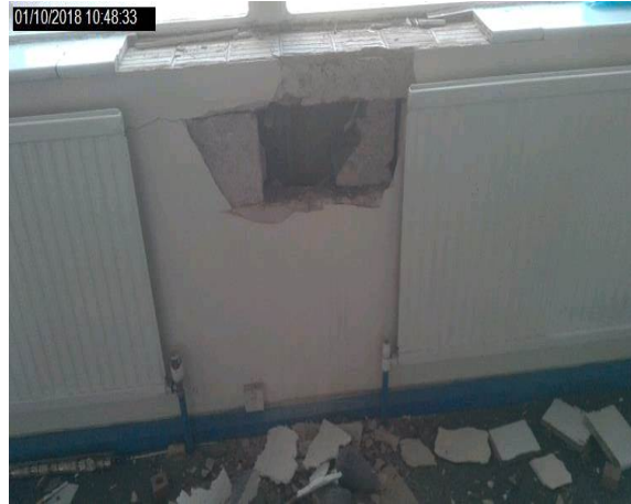
Intrusion 52 - Timber boxing to metal pipework
