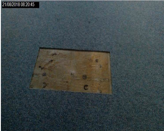
Intrusion 07 - Low level timber panels to wall void heaters
