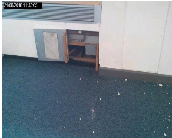
Intrusion 20 - Plaster to plasterboard to glass fibre insulation to timber panel
