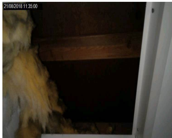
Intrusion 20 - Plaster to plasterboard to glass fibre insulation to timber panel
