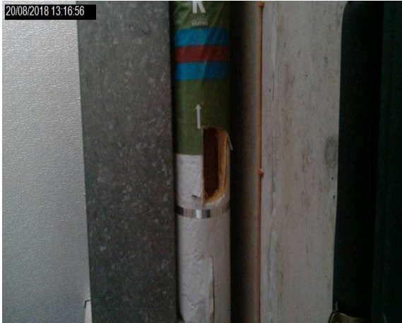
Intrusion 03 - Plaster to plasterboard to glass fibre insulation to timber panel
