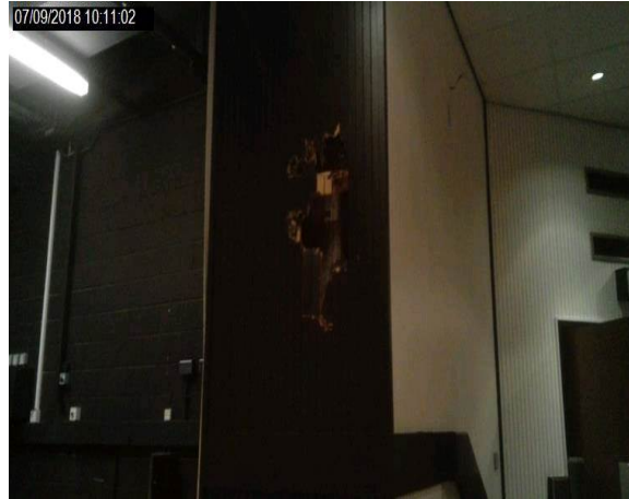
Intrusion 56 - Insulating board panel to rear of redundant door
