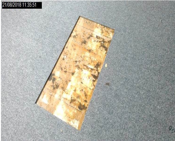
Intrusion 23 - Compressed fibre suspended tiles to textured coating
