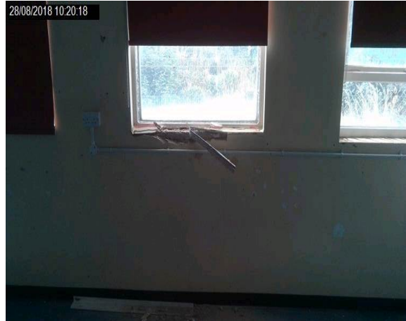
Intrusion 04 - Into brick wall beneath window
