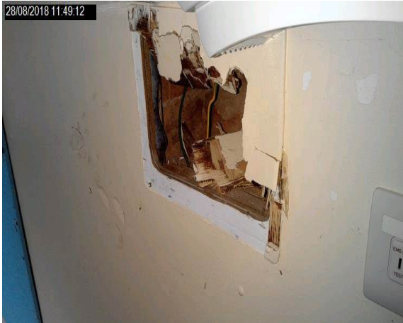
Intrusion 11 - Timber boxing to metal pipework
