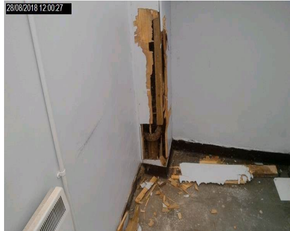
Intrusion 12 - Timber boxing to sliding door mechanism
