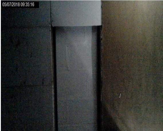
Intrusion 03 - Ply lining to polystyrene to block
