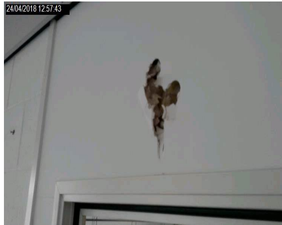
Intrusion 12 - Plasterboard door header to glass fibre insulation cavity
