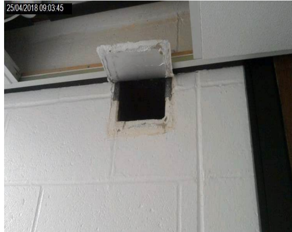
Intrusion 20 - Timber panel to secondary timber panel to heater wall void
