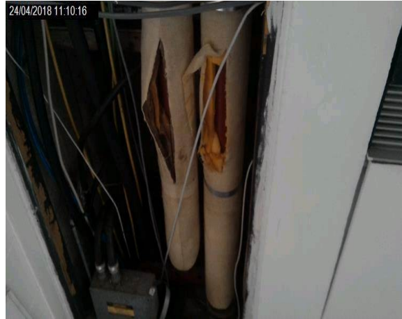
Intrusion 04 - Glass fibre insulation to metal pipework
