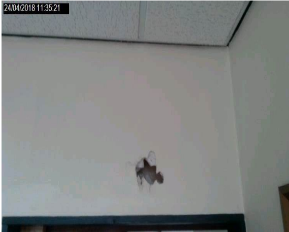
Intrusion 07 - Fibreglass panel to foam insulation to timber panel to riser
