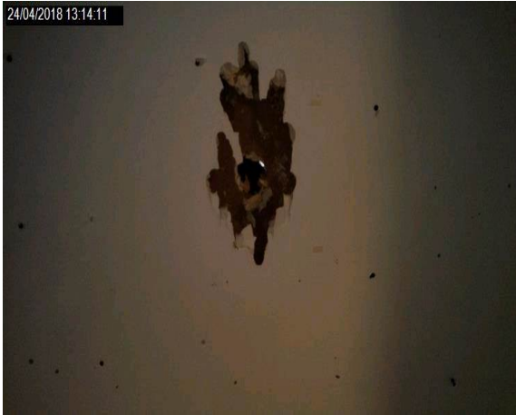
Intrusion 15 - Block wall to ventilation riser room 3.33A
