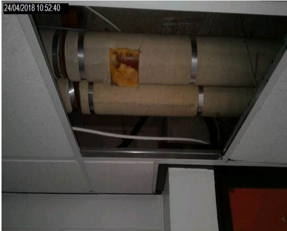
Intrusion 03 - Glass fibre insulation to metal pipework
