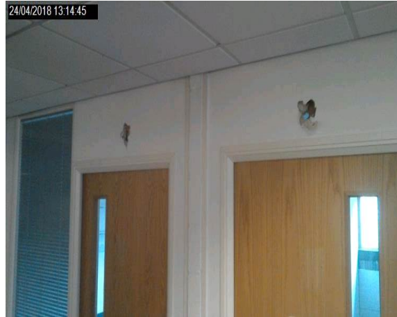
Intrusion 16 - Fibreglass panel to riser
