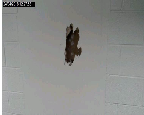
Intrusion 12 - Plasterboard door header to glass fibre insulation cavity
