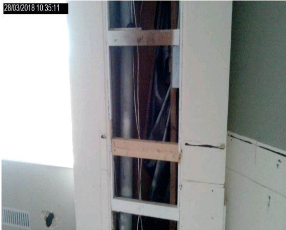
Intrusion 03 - Plaster to plasterboard to textured coating
