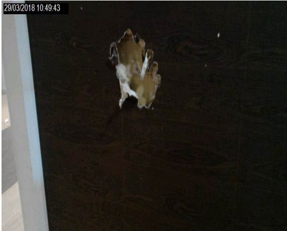
Intrusion 039 - Metal sheet to foam to metal external sheet roof covering
