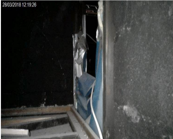
Intrusion 027 - Plastic surround to air vent
