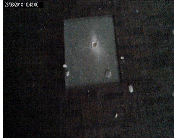
Intrusion 020 - Plaster to plasterboard to concrete
