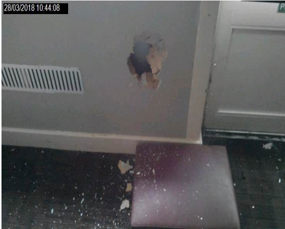
Intrusion 015 - Timber panel to riser, insulating board top panel, plasterboard to glazing, plaster to plasterboard ceiling to textured coating
