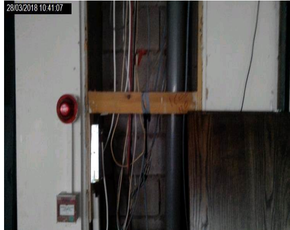
Intrusion 012 - Timber panels to pre cast concrete riser, cloth wrap glass fibre insulation to metal pipework, insulating board panel top panel
