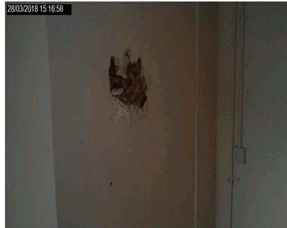
Intrusion 032 - Plasterboard to concrete pillar
