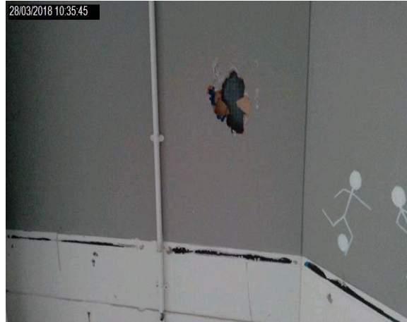
Intrusion 04 - Plaster to plasterboard glass fibre
