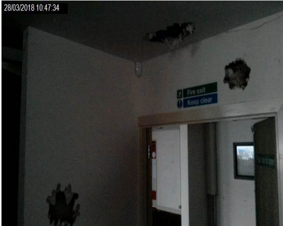
Intrusion 019 - Plaster to plasterboard to timber
