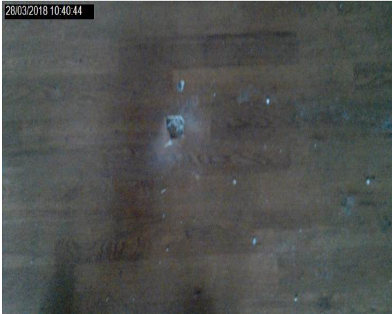
Intrusion 011 - Plaster to plasterboard to textured coating to concrete
