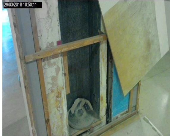
Intrusion 040 - Metal grate to heating pipes polystyrene behind to steel joists
