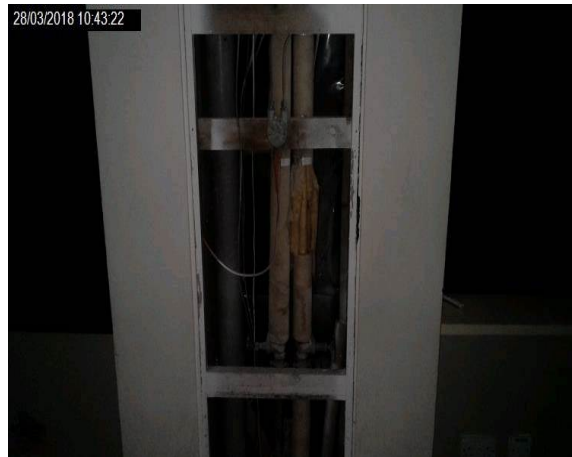
Intrusion 012 - Timber panels to pre cast concrete riser, cloth wrap glass fibre insulation to metal pipework, insulating board panel top panel
