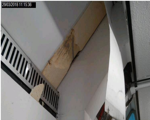
Intrusion 039 - Metal sheet to foam to metal external sheet roof covering
