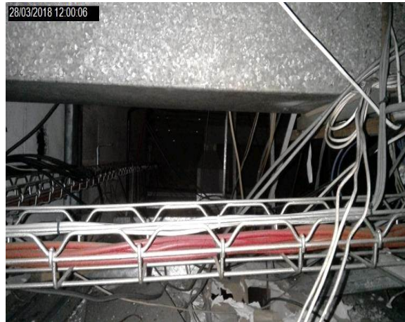
Intrusion 024 - Insulating board panel over female toilets first entrance door
