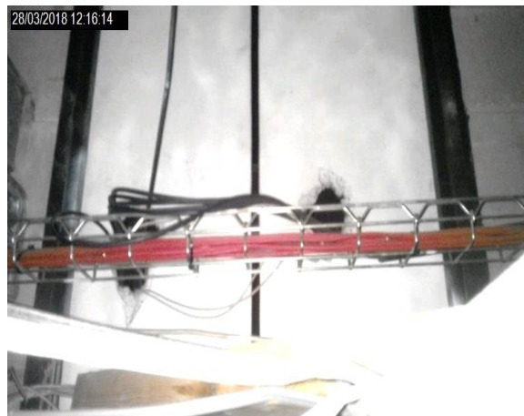
Intrusion 024 - Insulating board panel over female toilets first entrance door
