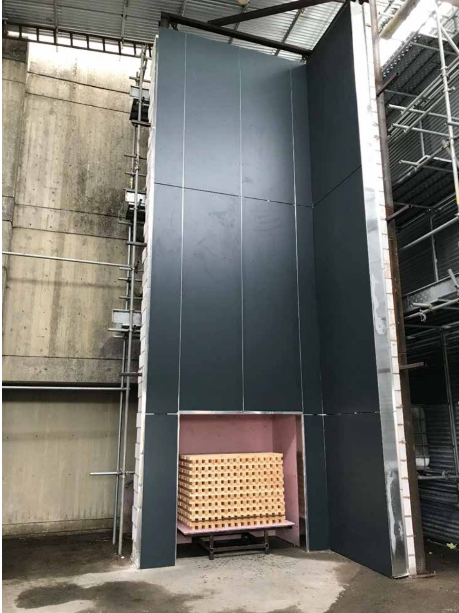
Figure 2 – Finished installation of cladding system under test
