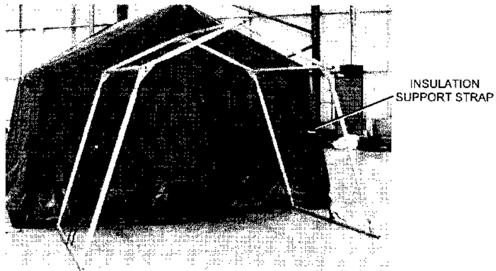
Fig 18 Frame with insulation support strap
