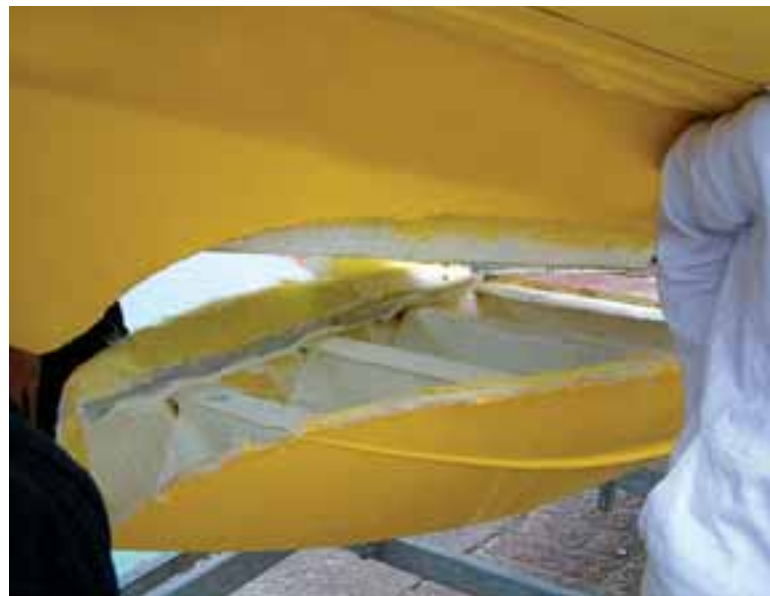
Figure 3 – Hull lifted to expose split
