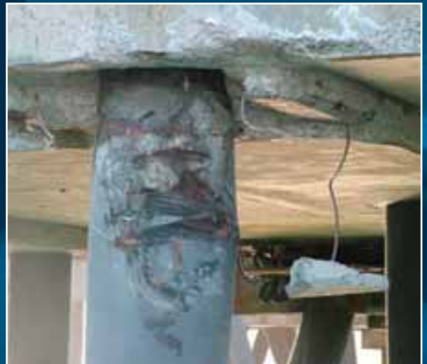
Figure 3: Damage to the jetty
