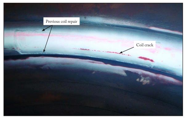
Figure 2: Port thermal oil heater coil fracture
