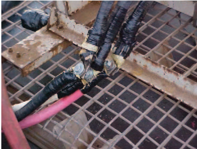
Figure 2: Shore services supply cable
