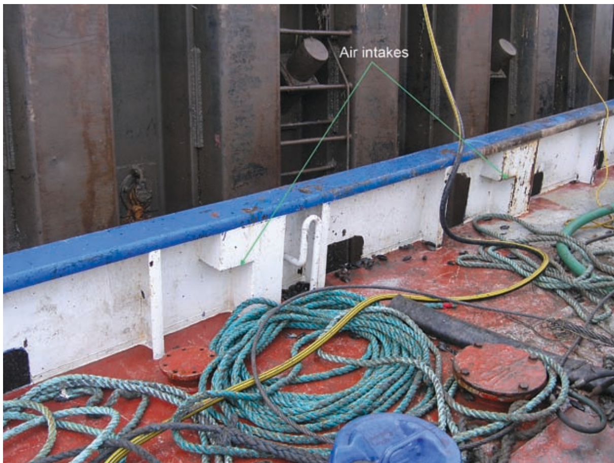
Figure 1: Deck, showing engine room air intakes
