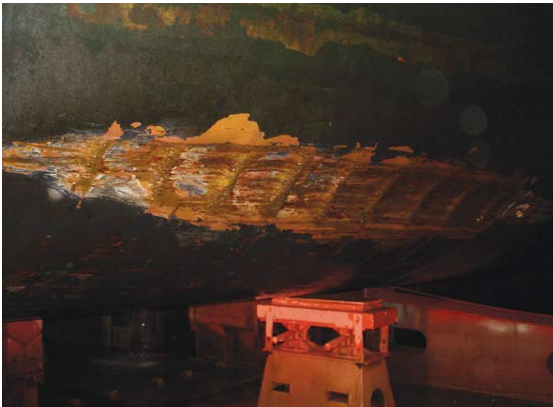
Damage below the waterline
