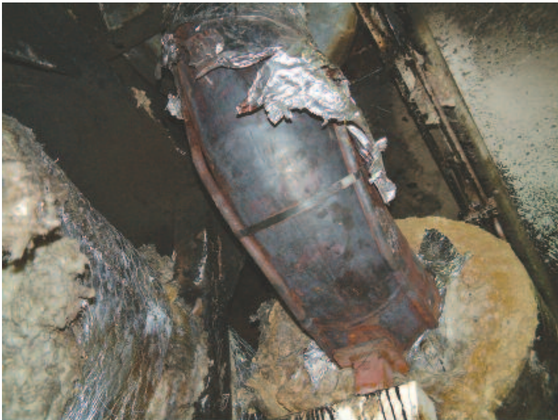
Bitumen pipe with lagging removed
