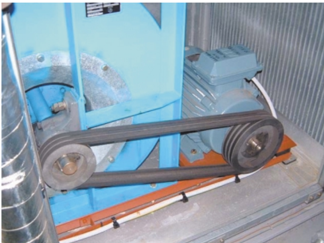
Figure 2: Motor fan unit and vee belts
