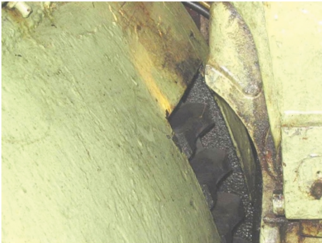
The gap between the turning gear's worm and the flywheel
