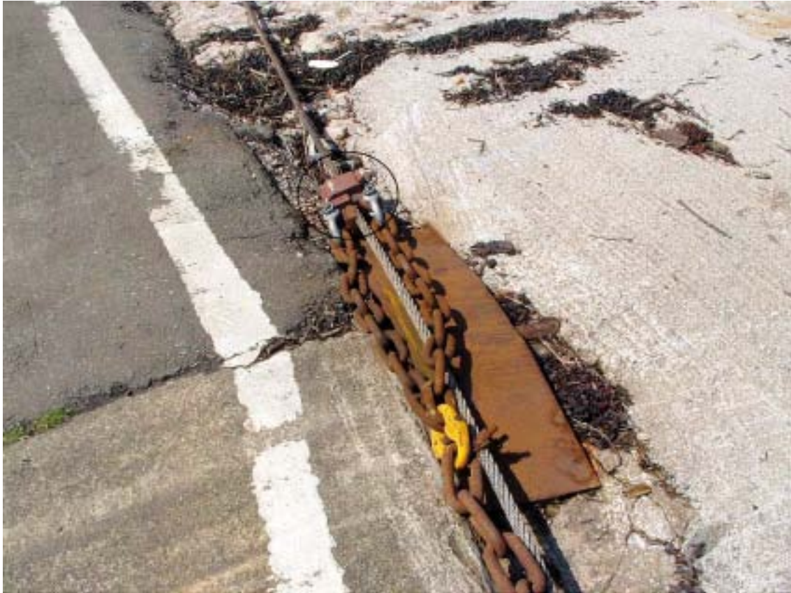
Figure 2 – Wire now attached to chain using carpenter's stopper
