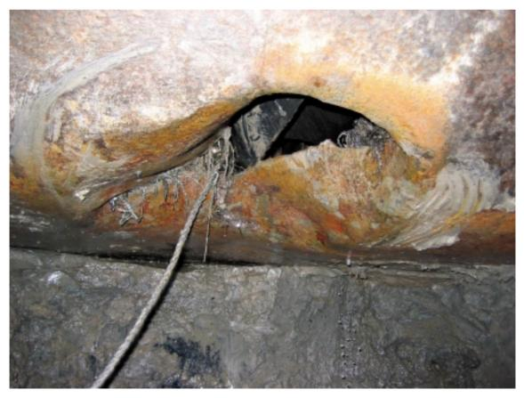
Photograph showing gash in single skin shell plating
