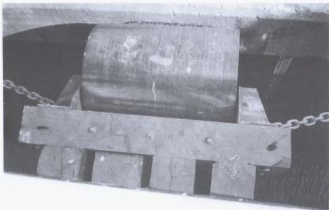
Photograph 3 Quay pile with fender
