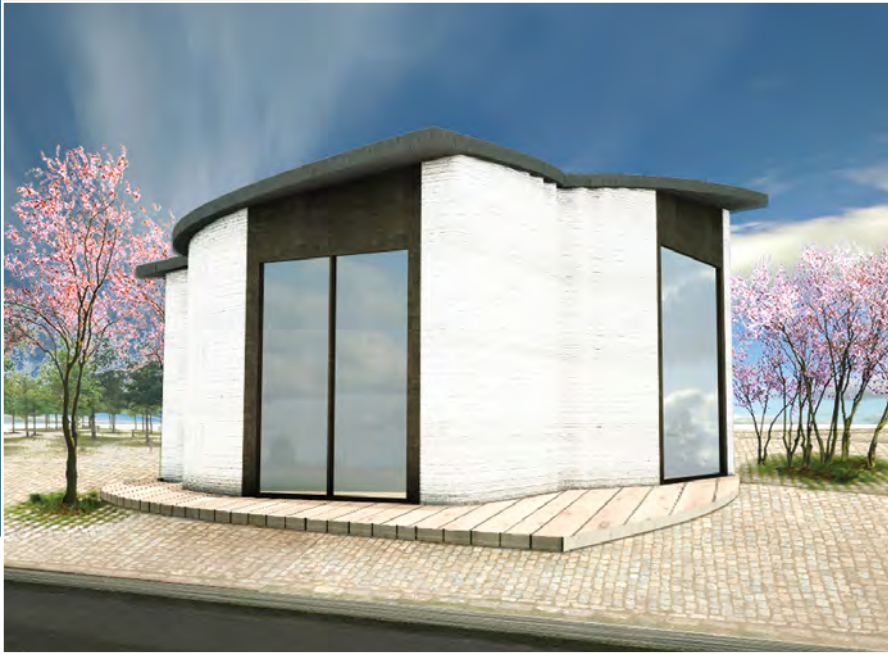
A Danish 3D printed building (walls and foundations): the first in Europe. Known as BOD (Building On Demand)
