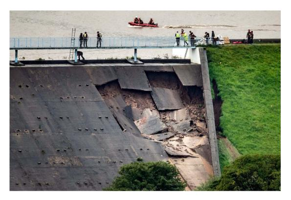
Figure 7. The Final Stage of Collapse of Panels. Note the undermining of the lefthand chute wall.
