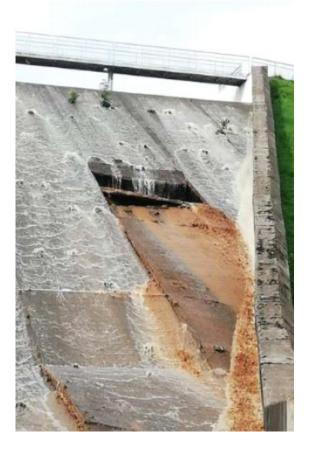
Figure 5. Collapse of the First Slab into the Void (note the slabs that have been pushed up towards the foot of the spillway chute).
