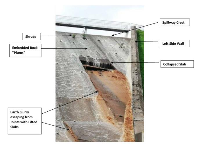
Figure. B2 The initial slab collapse
