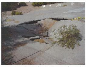
Figure 4.—Structural collapse of the slab system occurs when enough undermining has occurred to cause loss of support. This damage is typical of slabs placed on soil foundations (note: this slab is not reinforced so failure is more evident).
