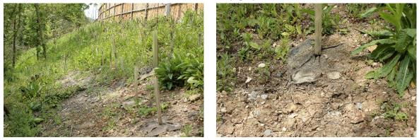
Figure 5-6 The planting plot adjacent to the clockwise carriageway directly west of Woodgreen Road Underbridge with construction debris and soil heaped up around the base of a retained tree (left), and evidence of minimal topsoil (right).
