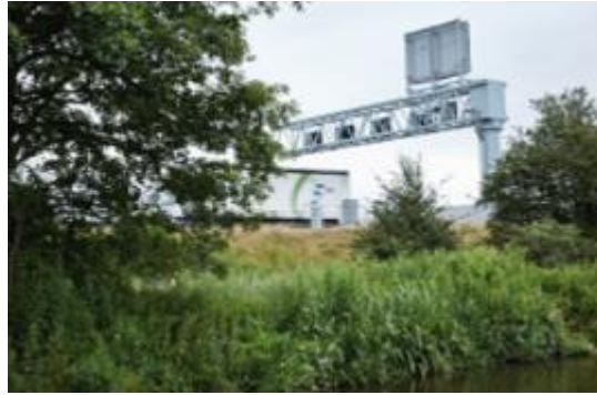
Figure 5-5 Lack of tree planting
