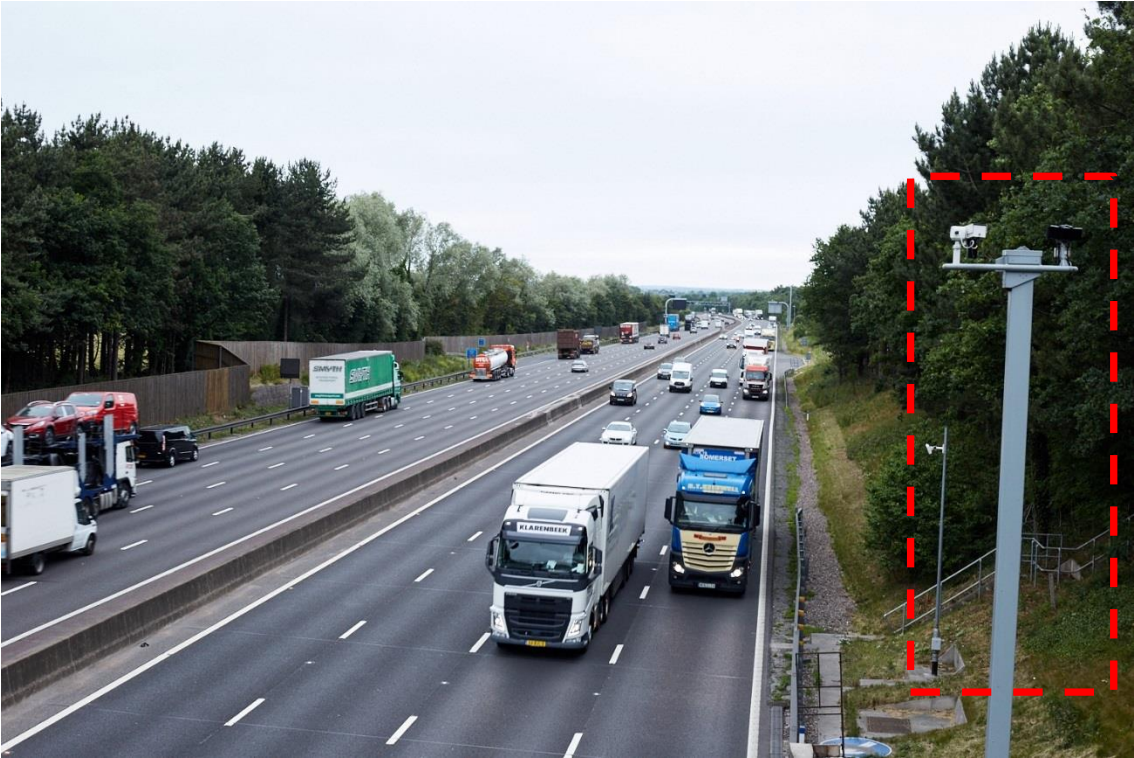
Figure 3-5 Additional CCTV cameras and emergency refuge areas
